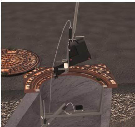
Using the Mounting-hook the trap is lowered down the manhole.
